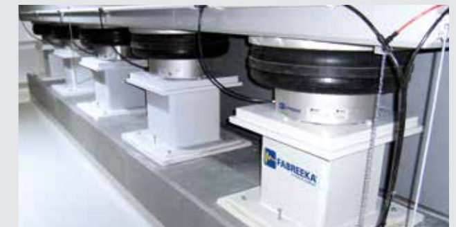
BMW test bench bearing
