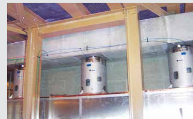
Measuring machine foundation
