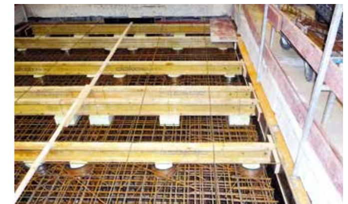
Support foundation rebar
