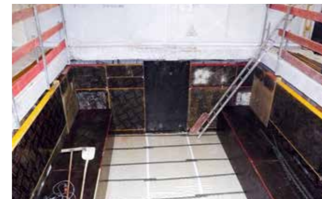
Formwork on the support foundation
